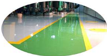
Epoxy Floor Coating
